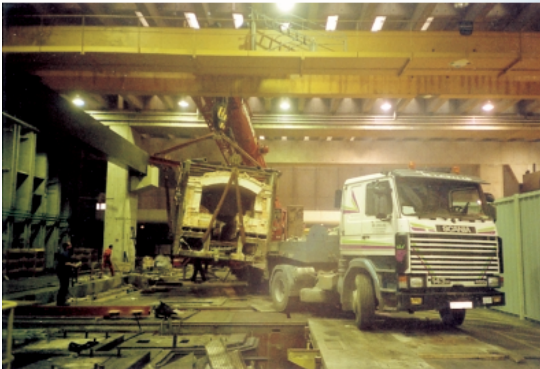
Disassembling a rolling mill and a furnace in Monnaie de Paris (Bordeaux).
